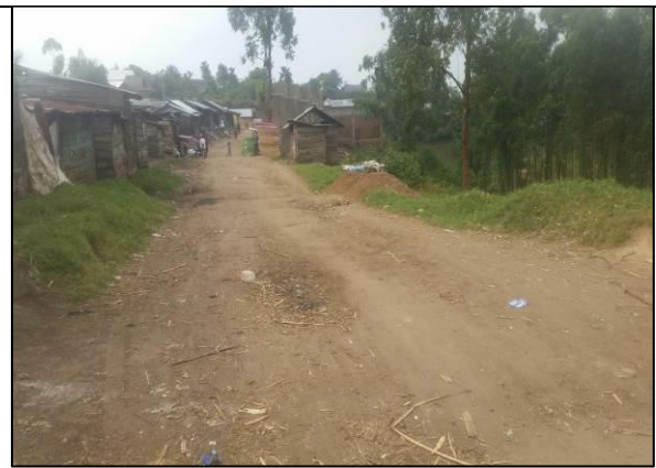
Access road around the market
