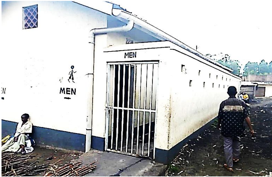
Figure 5: Pit latrine at Lhubiriha Market
