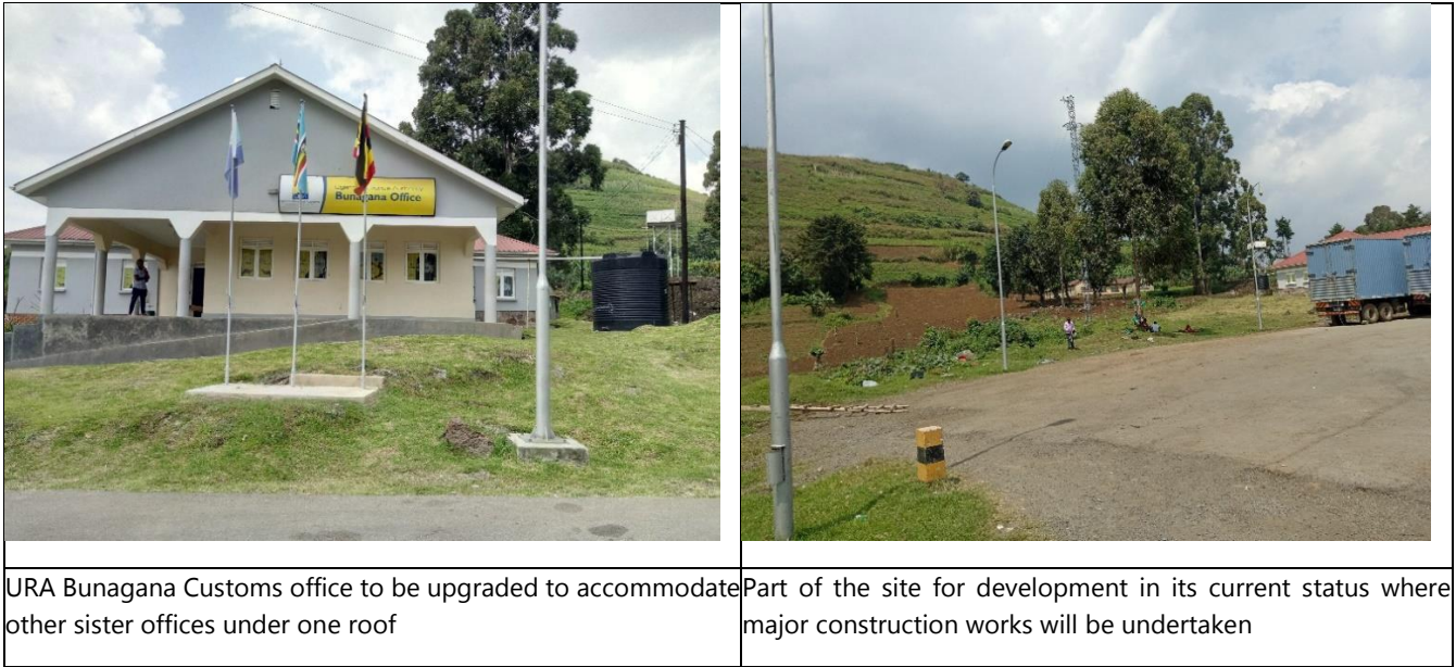
Figure 2: Photographs Portraying Project Site Current Status
